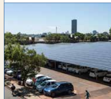
Clean Energy Initiatives
