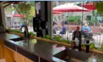
Kitchens provide boiling & chilled filtered water
